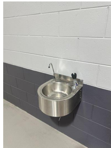
Photo of drinking fountain along walkway juts out from wall, although colour contrast is present. There is no tactile (inc. Braille) signage.
