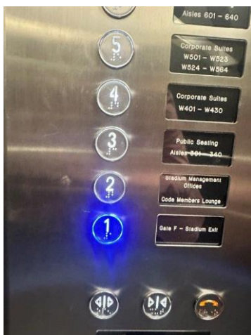
Photo of tactile (inc. Braille) internal lift buttons
