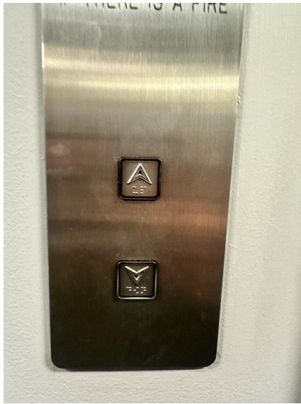
Photo of tactile (inc. Braille) lift buttons
