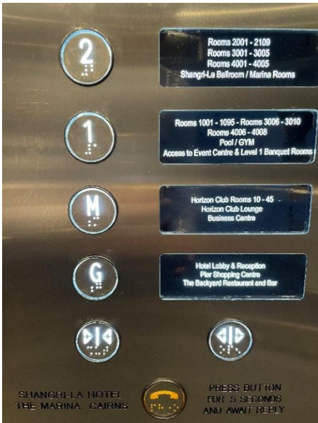
Photo of elevators with Braille
