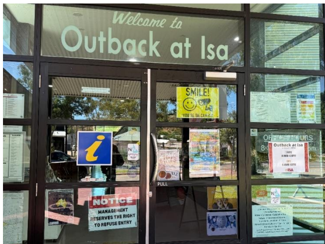
Photo showing it is unclear where the entry way is
