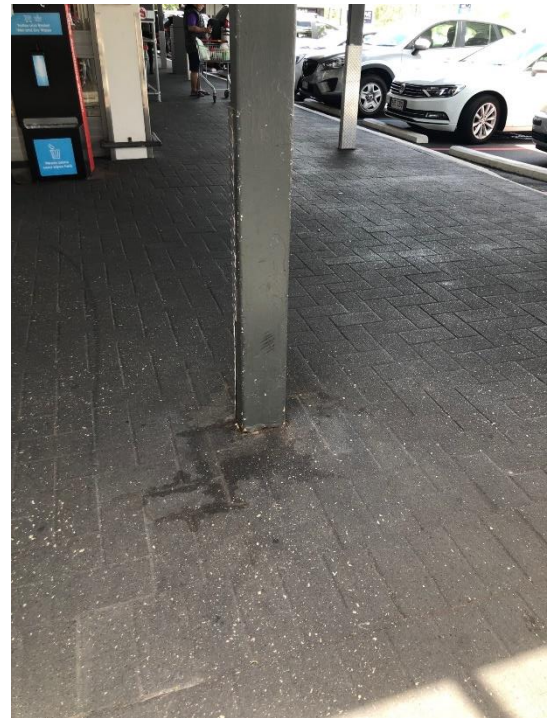
No colour-contrast between post and floor surface.
