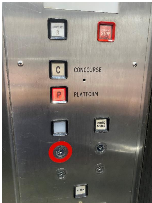
Unsupportive lift signage
