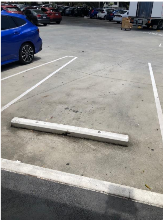
No contrast between concrete wheel stop or curb, and the carpark surface.
