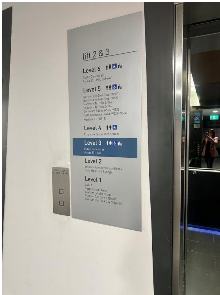
Braille signage outside lift is very extensive, however due to the amount of information and the formatting of the sign, is not height friendly for hands to read Braille.
