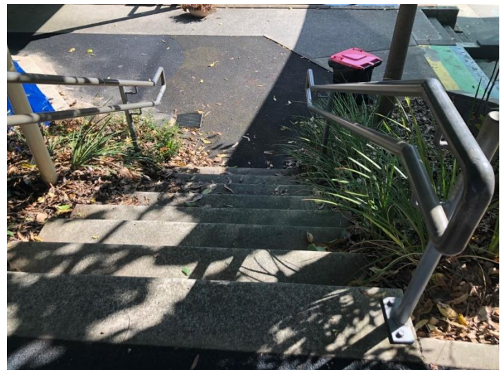
No colour-contrast between post and floor surface.
