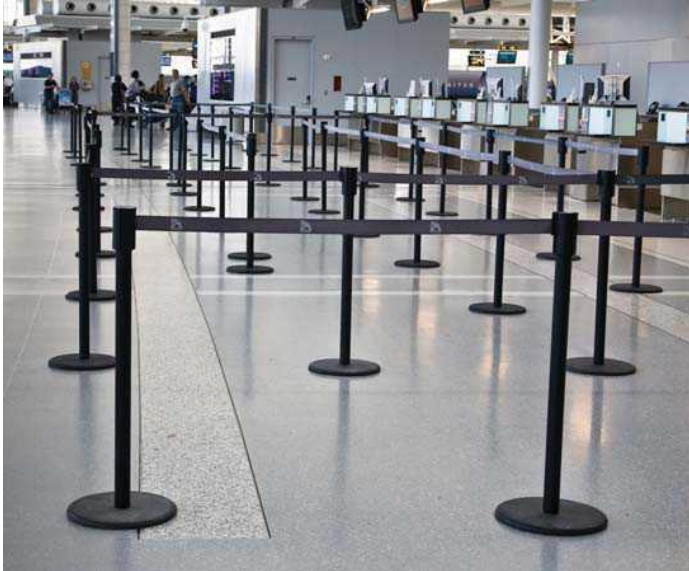
An example of a poor queuing system that projects into the space's main path of travel. However, the system illustrates good colour contrast to the surrounding floor surface.
