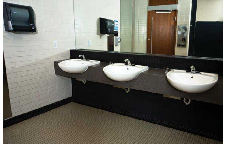
Good colour contrast in a public toilet
