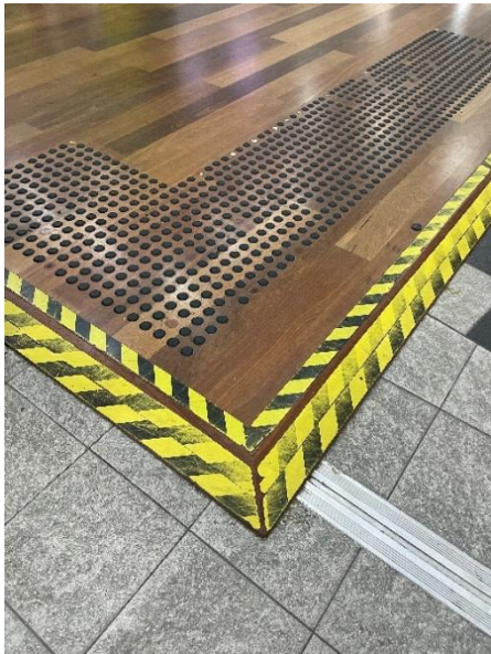
Elevated floor with hi-vis marking
