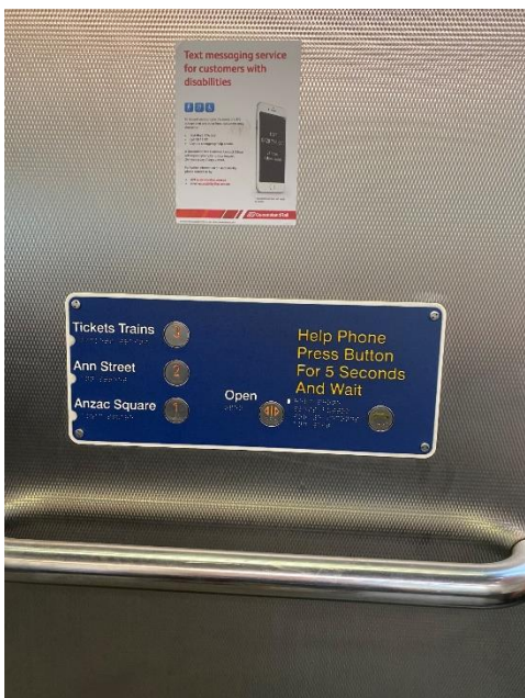
Supportive lift signage and handrail
