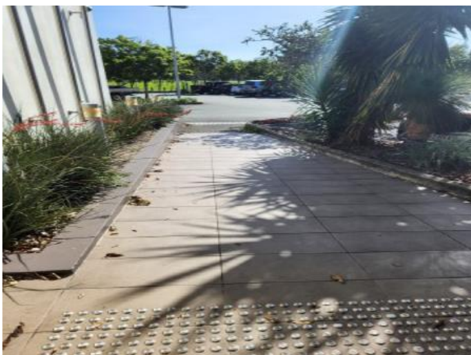
Photo of function area entrance – Tactile ground surface indicators
