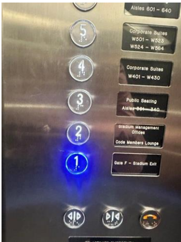
Tactile (inc. Braille) internal lift buttons
